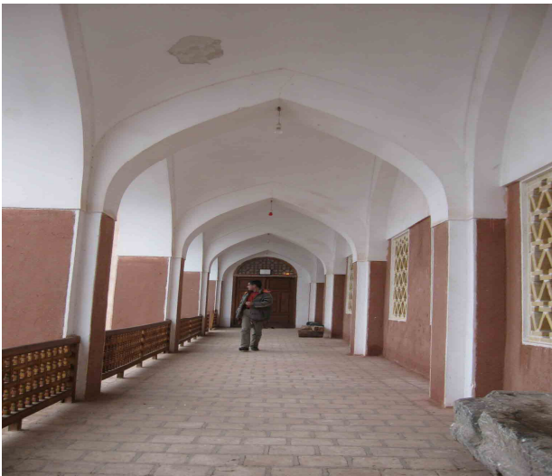
Fig. 5 Locating the wide, long and lofty balconies in the direction of the main seraglio entryway or in three or even in four sides of it
