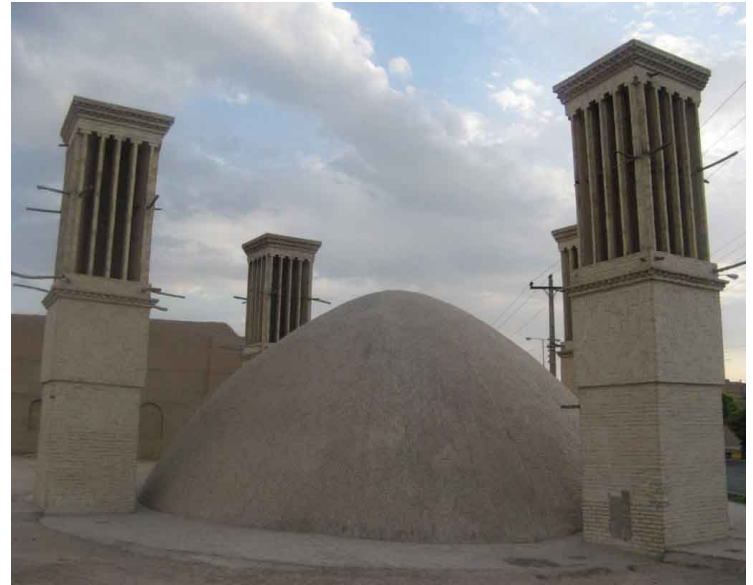
Fig. 2 the way of using arched-shaped ceiling in the air holes (Yazd, Iran)
