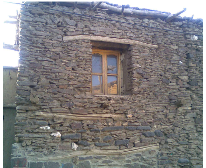
Fig. 3 using the stony thick wall in order to make the thermal insulator (Varkaneh village, Hamedan, Iran)
