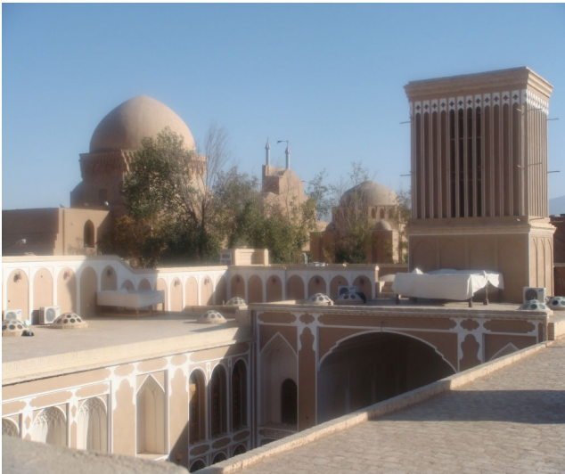
Fig. 1 The way of yard position in the centre and using the air hole (Yazd, Iran)
