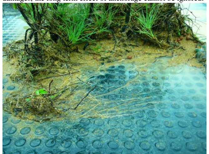
Fig. 8 Roots left on the membrane after some erosion; the plants are removed whereas roots which have anchored on the membrane are cut from the plant
