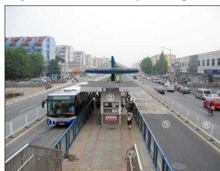
1 Advanced vehicle 2 Enhanced station 3 Off-board fare collection 4 Screen door system 5 Exclusive busway 6 Barrier 7 Overpass Fig. 4 Beijing Southern Axis BRT line 1
