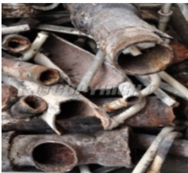
Fig. 16 Rusty broken pipes
